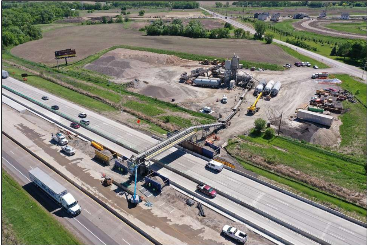
Concrete conveyor used on the I-94 Design-Build Project, Rogers to Maple Grove, MN (Source: C.S. McCrossan)
