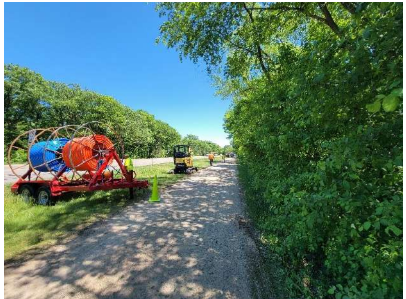
Fiber conduit installation in Minnetonka, Minnesota
