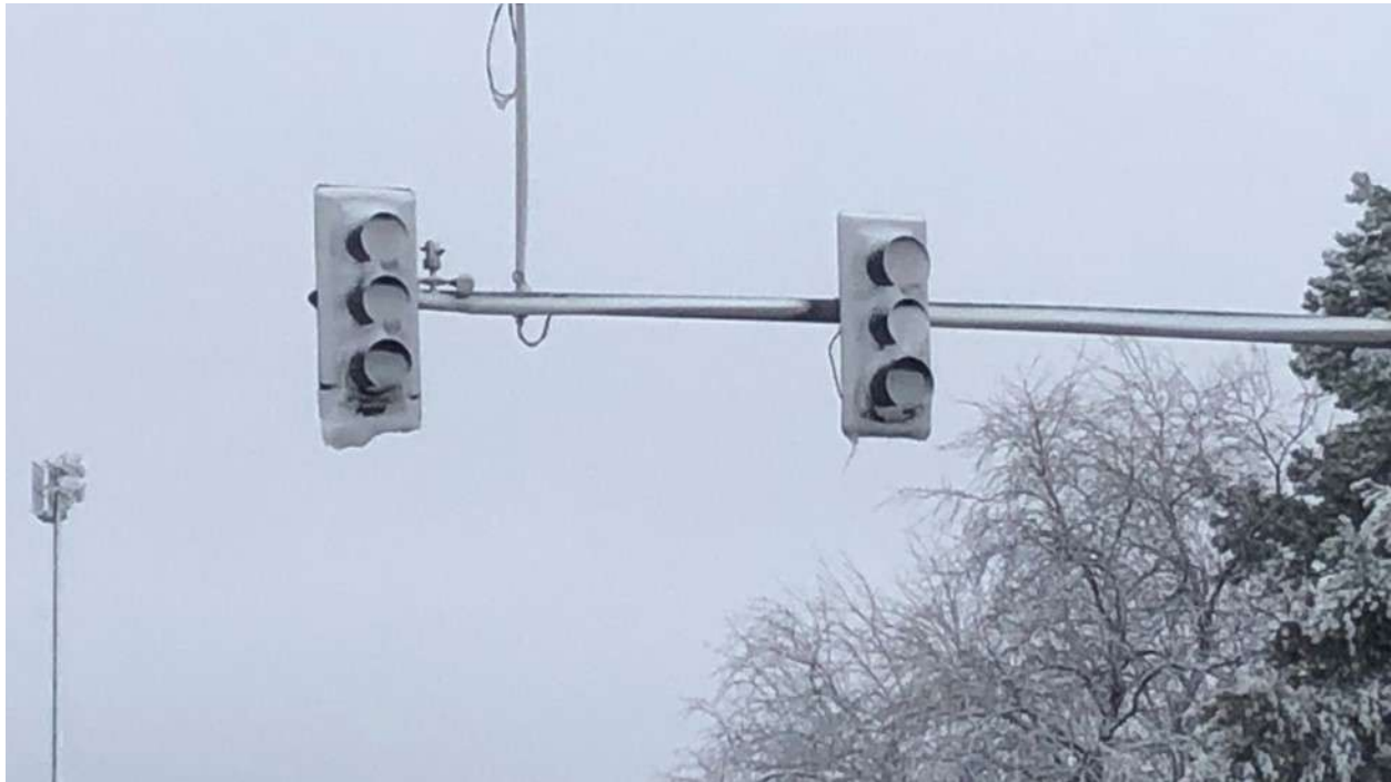
Snow Covered LED Signals. Source:
