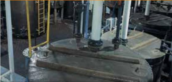
East Penn built the battery industry's first acid reclamation plant. The reclaimed acid is used in new batteries.
