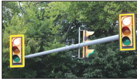
Exhibit 1: Retroreflective borders on backplates can provide a visual benefit during both daytime and nighttime conditions. (Source: VDOT)
