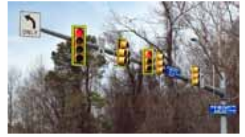
Reflective back plates increase traffic signal visibility at intersections
