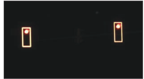
Exhibit 1: Retroreflective borders on backplates can provide a visual benefit during both daytime and nighttime conditions. (Source: VDOT)
